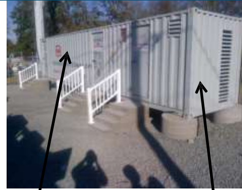
Inverter/Controls Integrated within one container
