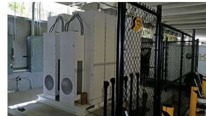
200 kW / 500 kWh Lithium Iron Phosphate - Charlotte, NC
