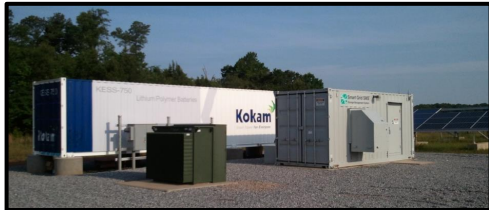
250 kW / 750 kWh Lithium Polymer - Charlotte, NC
