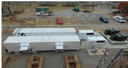
250 kW / 750 kWh Lithium Polymer - Charlotte, NC
