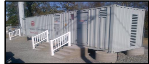
200 kW / 500 kWh Lithium Iron Phosphate - Charlotte, NC
