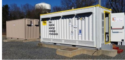
300 kW / 307 kWh Ultra Caps/Aquious Hybrid Ion - Mt. Holly, NC
